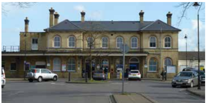
Bottom: The existing Victorian Station building
